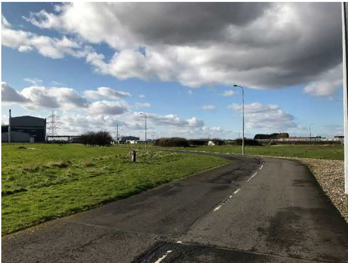
Photograph 6: Showing the Main Development Area of the Site with G10 – G17 in the background.
